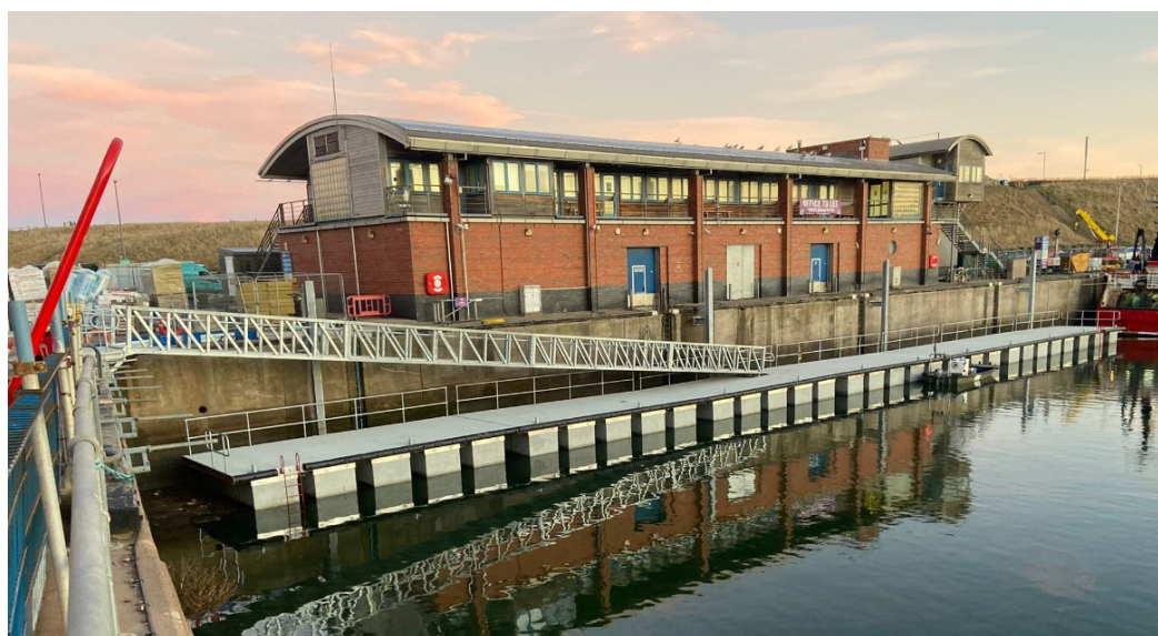
Figure 90 Typical floating pontoon and access gangway used for CTV operations (Source; Inland and Coastal Marina Systems)
