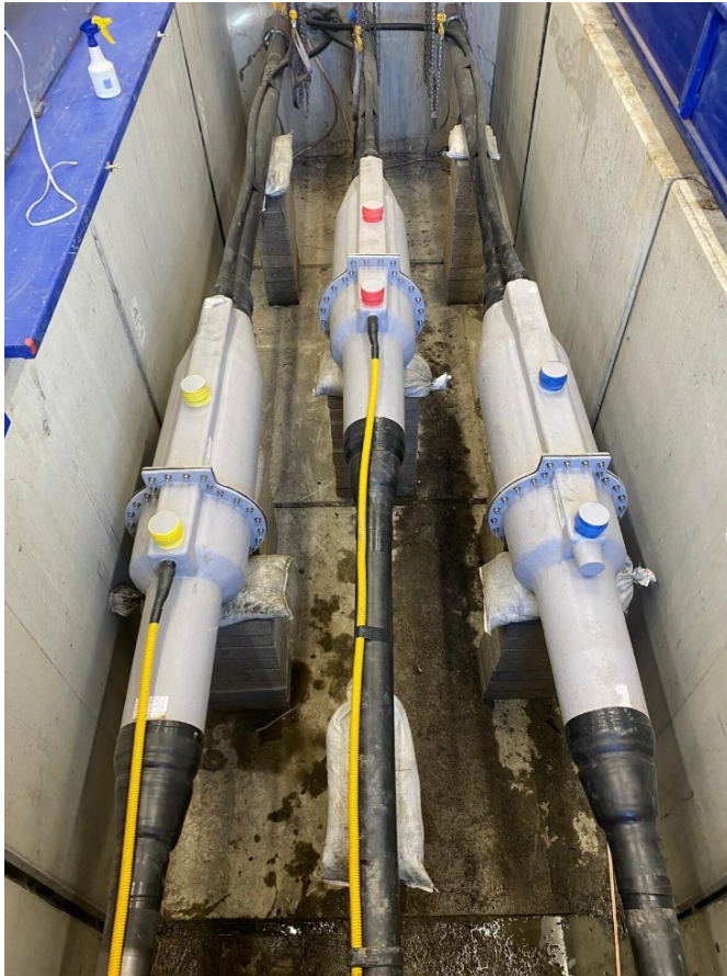
Figure 46 Example of HV cable joints in a concrete joint bay
