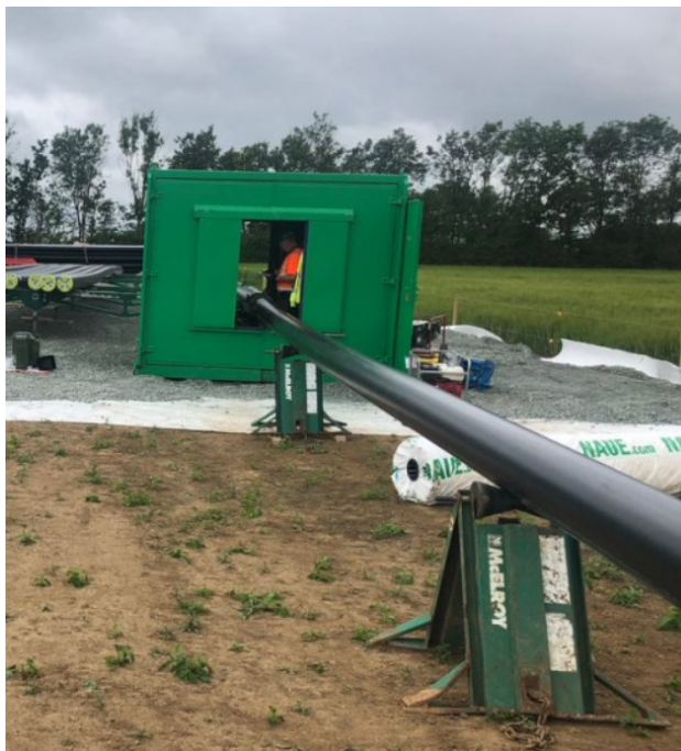
Figure 36 Example image of duct welding container (Source Stockton Drilling)
