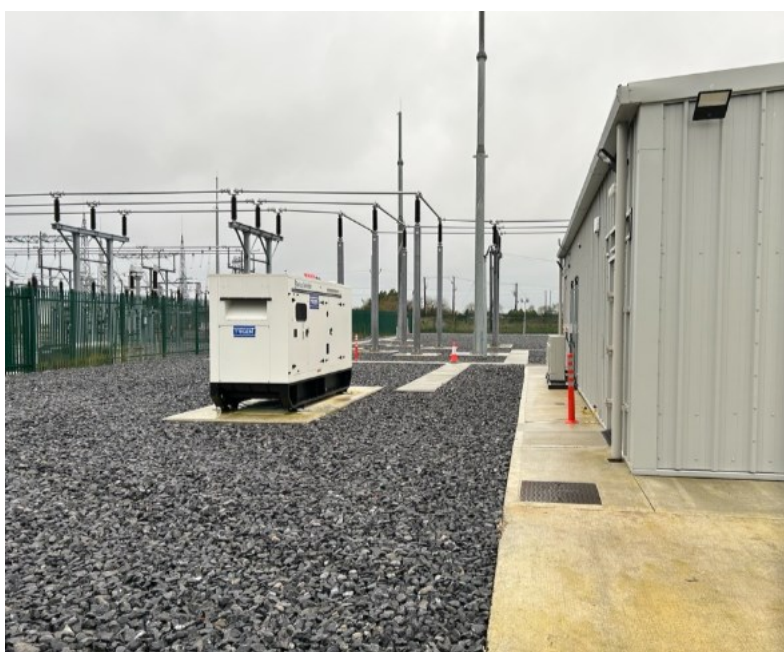
Figure 70 Example image of a back-up diesel generator beside a Statcom building
