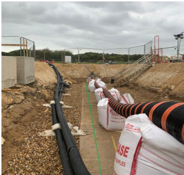
Figure 40 Example image of a typical TJB under construction with offshore export cable pulled in (right) and two link boxes, each with manholes for electrical and communication cable joints after reinstatement (left). (Source – RWE Renewables UK Ltd.)
