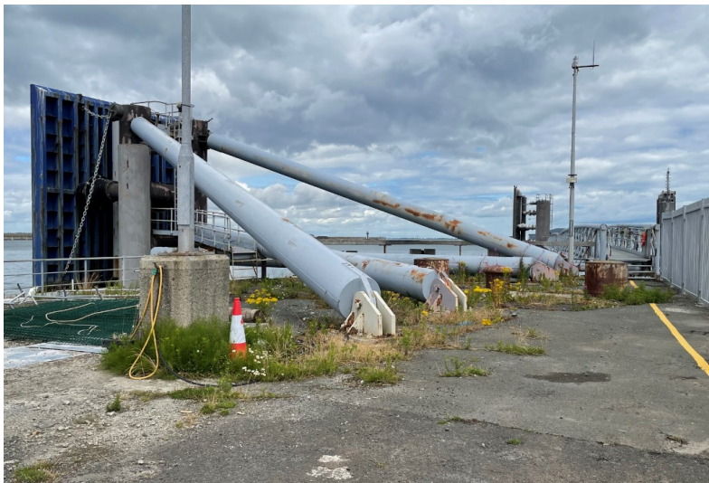
Figure 87 Existing fender structure and supporting steelwork at St. Michael's Pier
