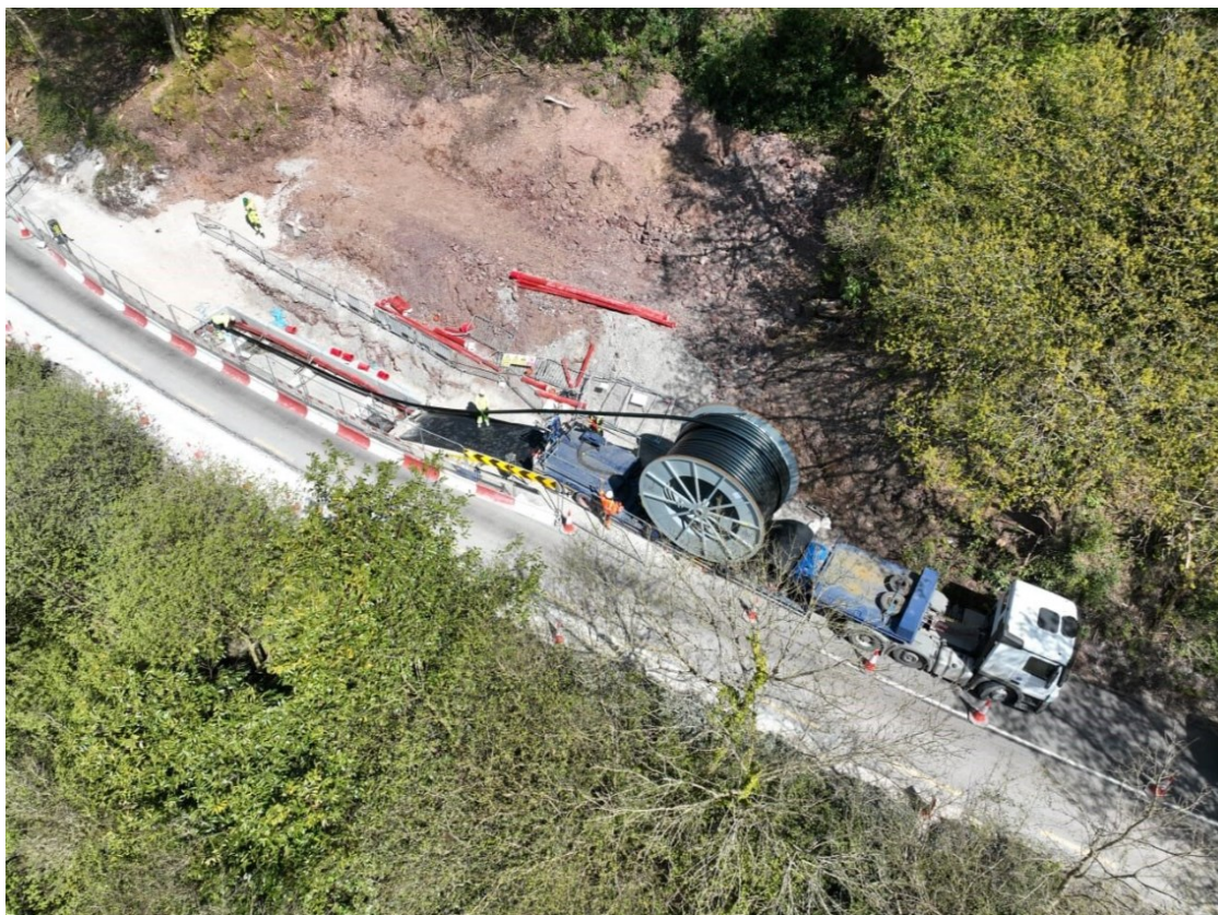
Figure 68 Example of a cable being pulled through a joint bay (source – Sorensens Civil Engineering - Celtic Interconnector)
