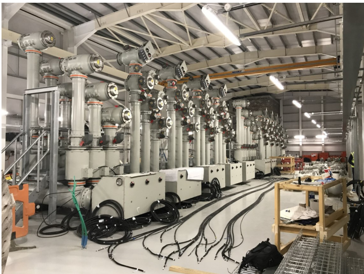
Figure 76 Example image equipment being installed inside the ground floor of a GIS Building
