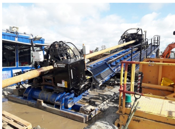
Figure 64 Example image of a typical HDD Rig set up (DD-440T) (Source J. Murphy & Sons Limited)
