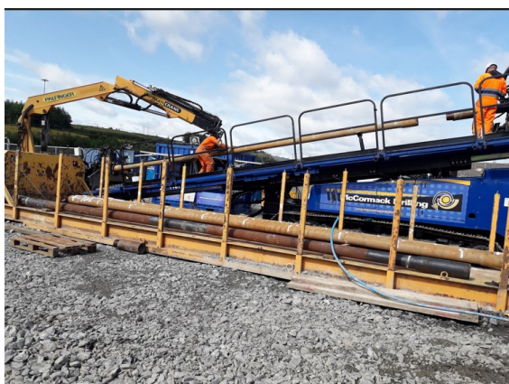
Figure 64 Example image of a typical HDD Rig set up (DD-440T) (Source J. Murphy & Sons Limited)
