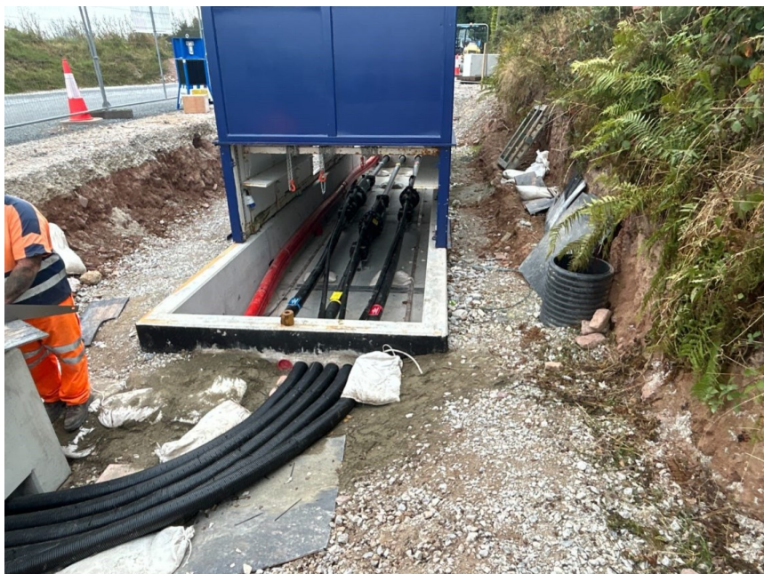
Figure 65 Example of transmission cables being installed at a joint bay (Source – Sorensens Civil Engineering - Celtic Interconnector)
