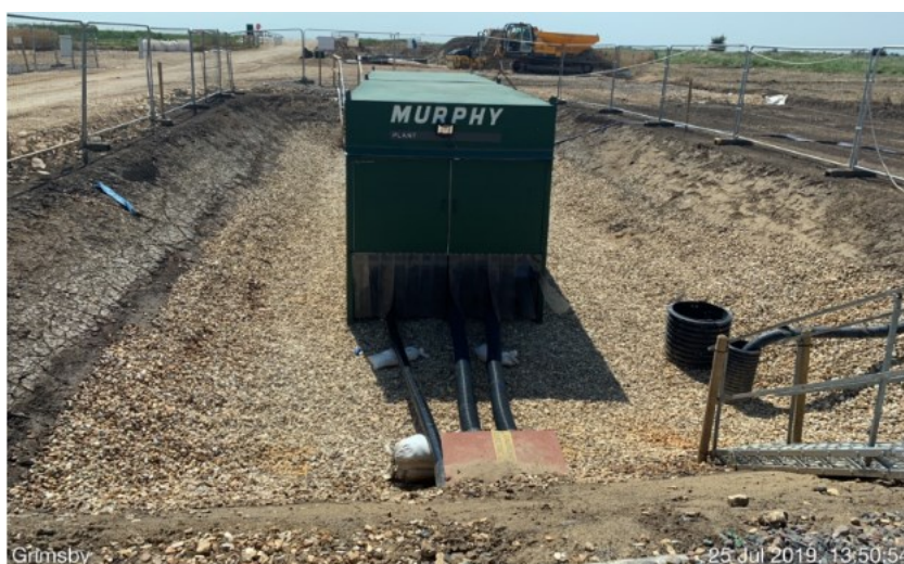
Figure 41 Example image of export cables being jointed in a controlled environment (Source – RWE Renewables UK Ltd.)
