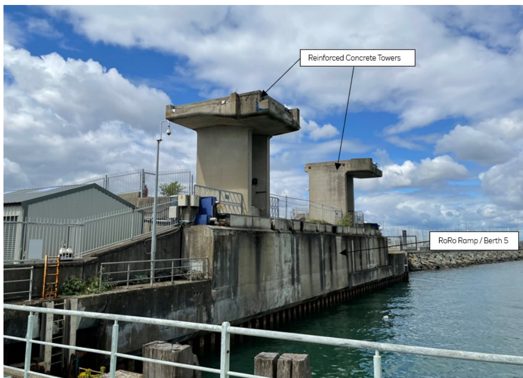
Figure 88 Existing RoRo ramp at Berth 5
