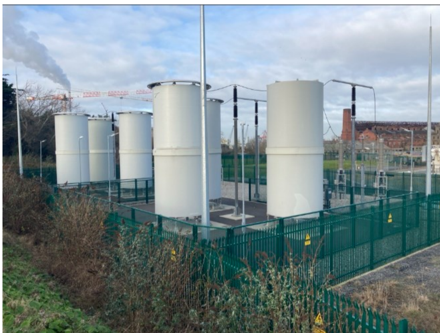
Figure 72 Example image of shunt reactors in an onshore substation compound, with lightning protection
