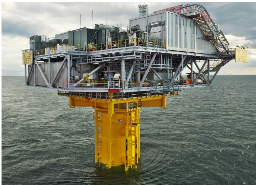
Figure 13 An example of an offshore substation platform on monopile foundation, Triton Knoll Offshore Wind Farm (RWE).
