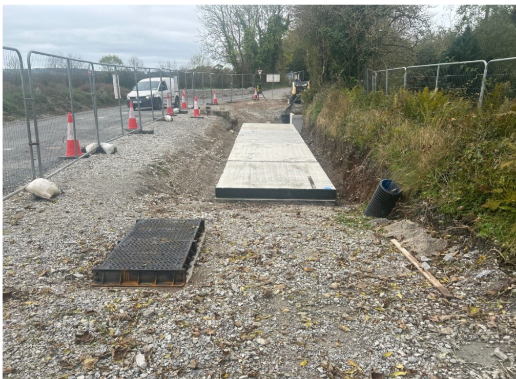
Figure 66 Example of a joint bay concrete lid with the manhole inspection cover for the communications chamber adjacent (Source – Sorensens Civil Engineering - Celtic Interconnector)
